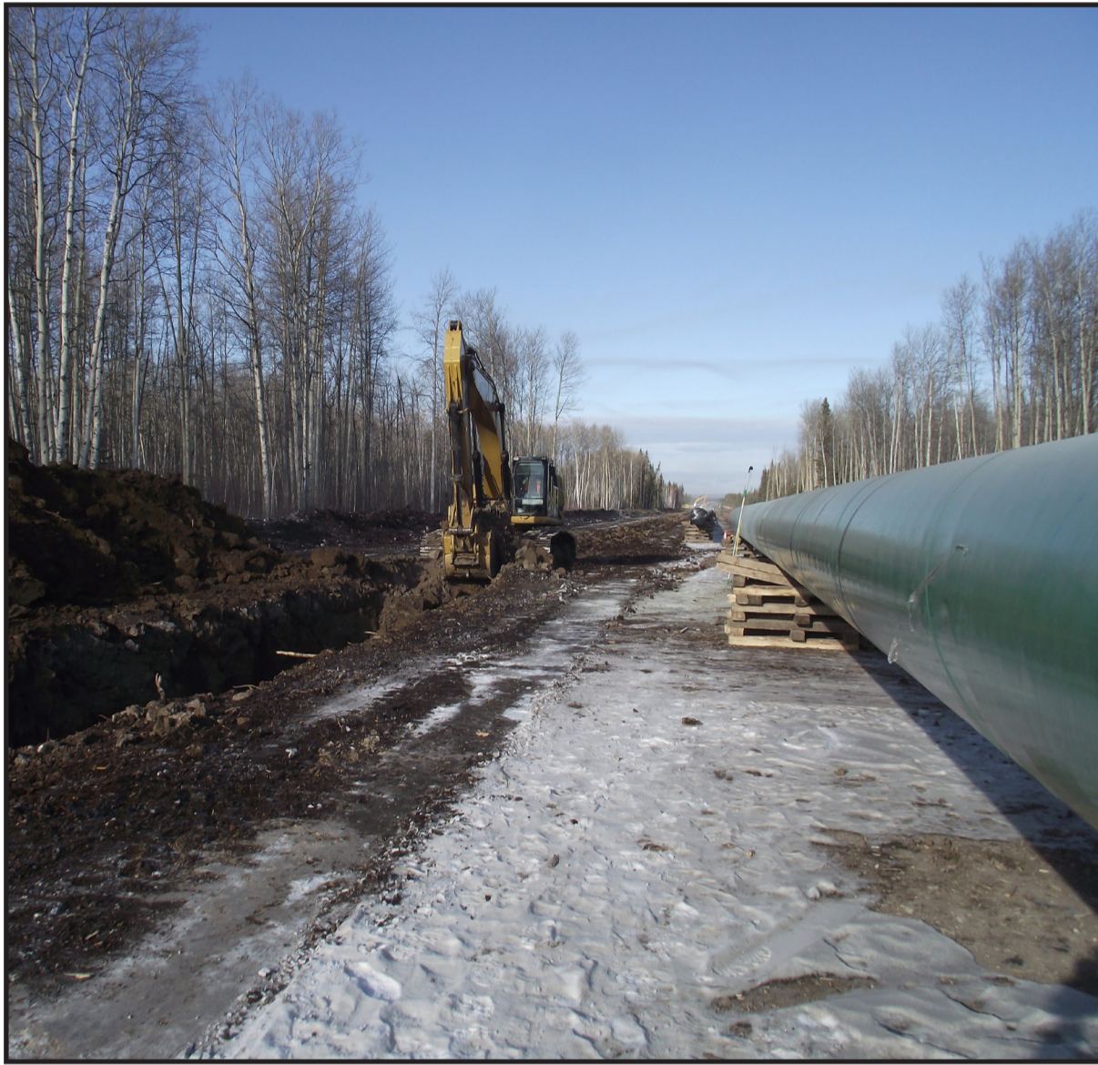
CCS requires pipes ... lots of them
