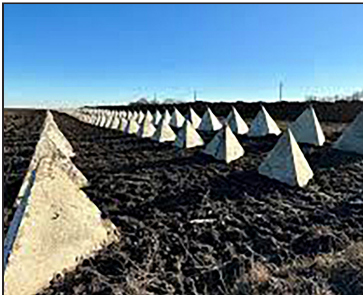
Russia has been putting in place fearsome defence systems, including rows of ‘dragons teeth’. Three or four feet high blocks of reinforced concrete, they are designed to stop or slow tanks and other military vehicles
